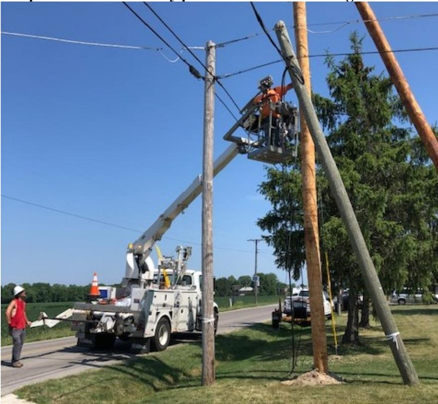
**New Lions Way Bentley path construction. Placement of new cable wire on new poles to make room for construction of pathway along Bentley Road between Richland Drive & Riley Street. It is anticipated the project will be completed in August 2020. Lion Dick Ramseyer**
